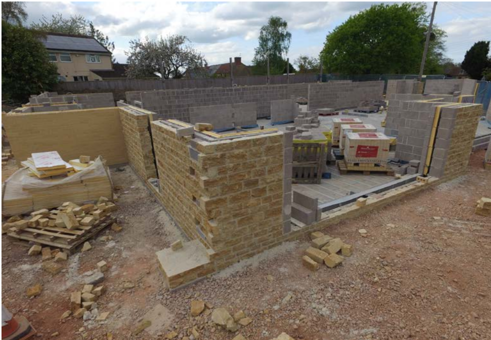
Photo 4 Showing stone and brick elevations
