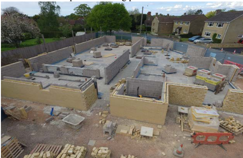
Photo 2. Showing brick and stone elevations
