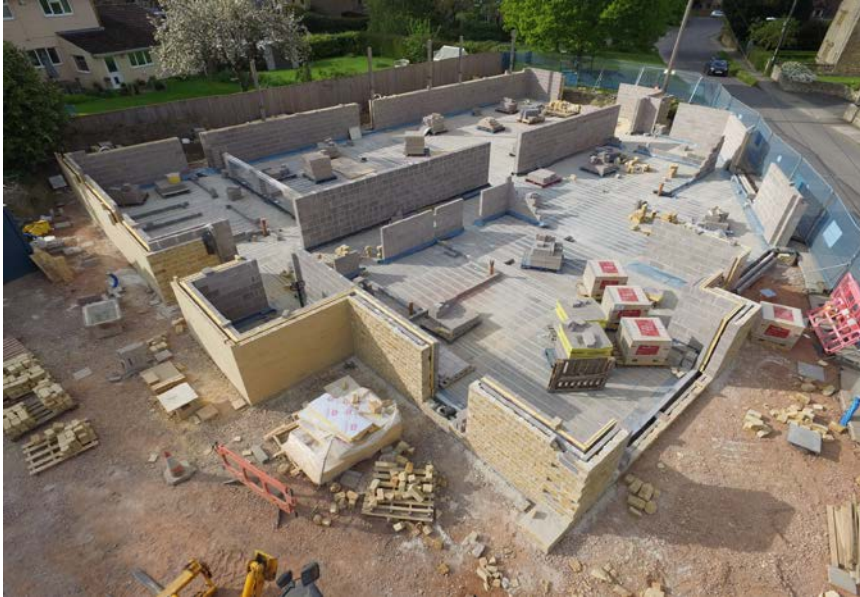
Photo. 3 View from above car park entrance looking across the site.
