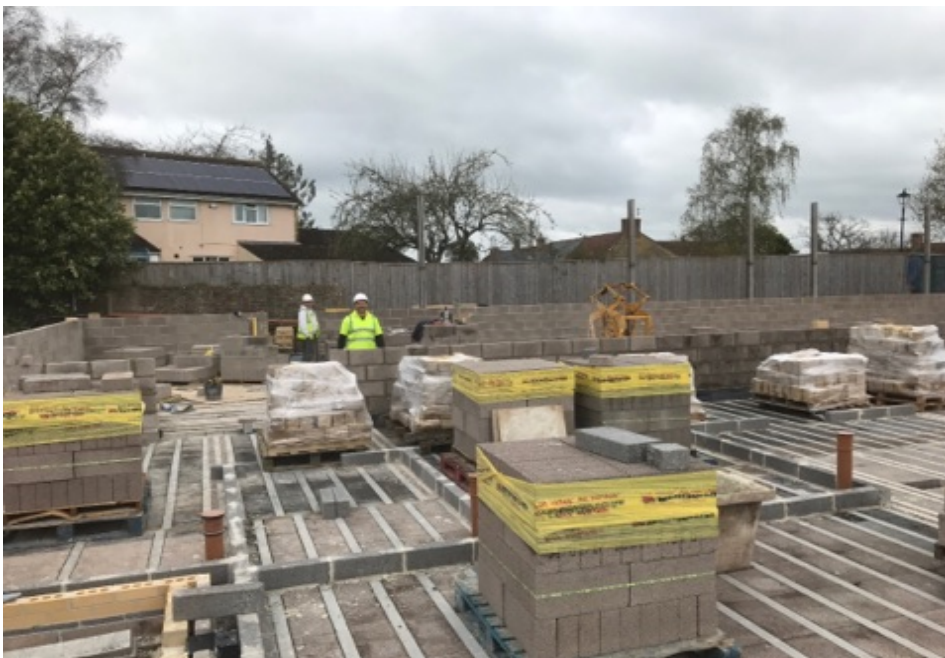
Photo 4 Masons building internal concrete block skin
