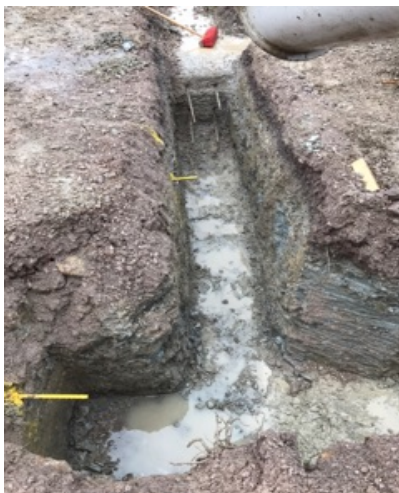
Photo 2. Last Foundation section being poured
