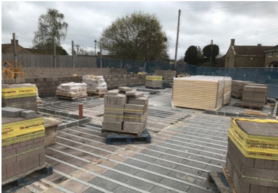
Photo. 3 Showing block & Beam installation wind posts to rear elevation & masonry
