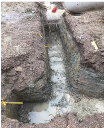
Photo 2. Last Foundation section being poured
