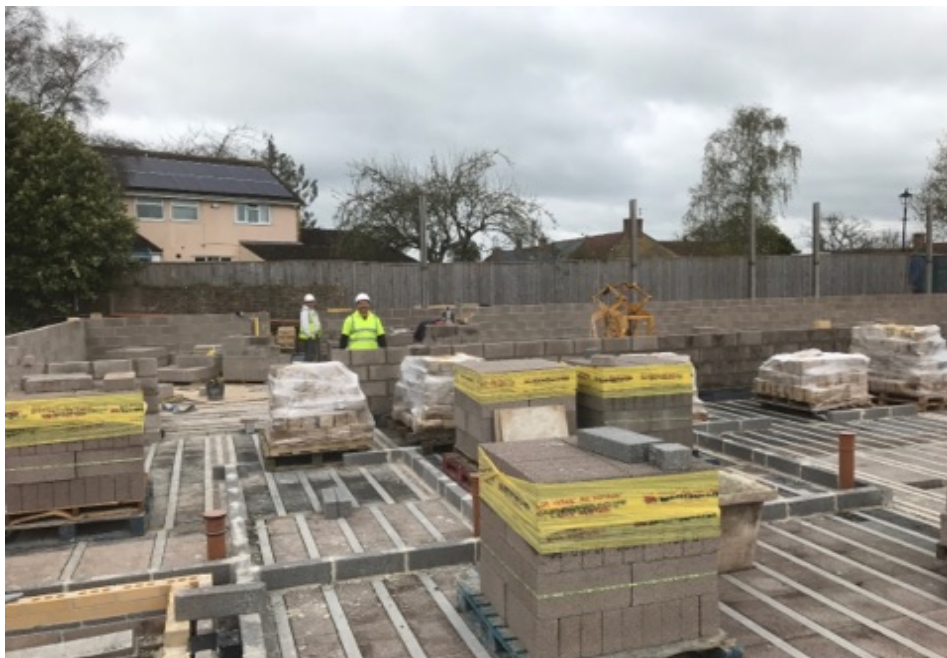
Photo 4 Masons building internal concrete block skin
