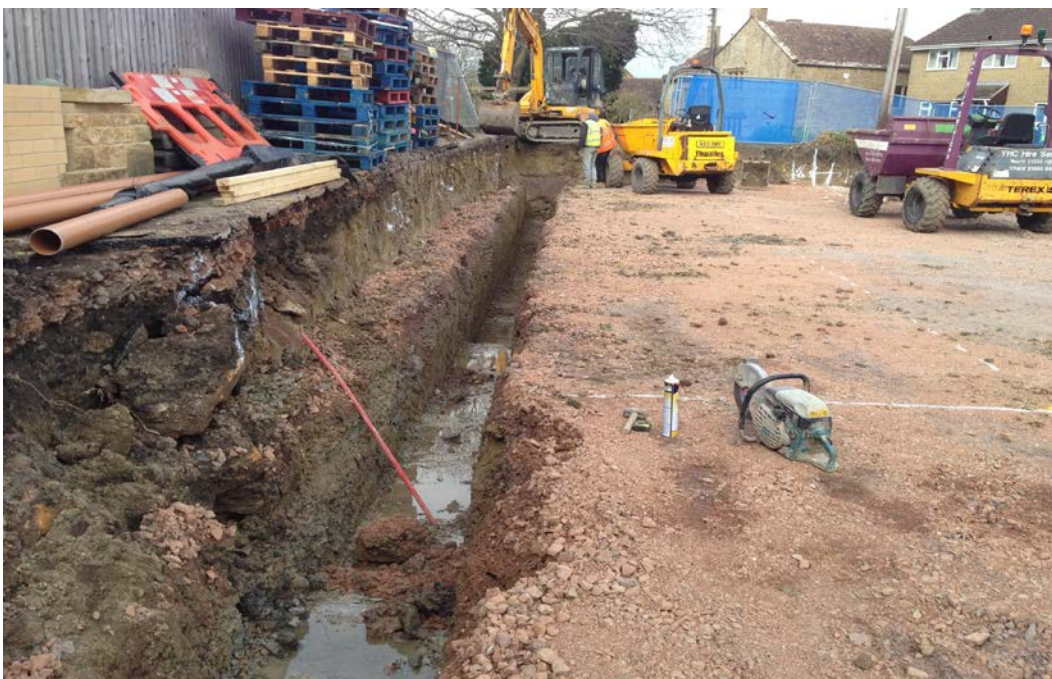
Photo 2. Foundation Excavations
