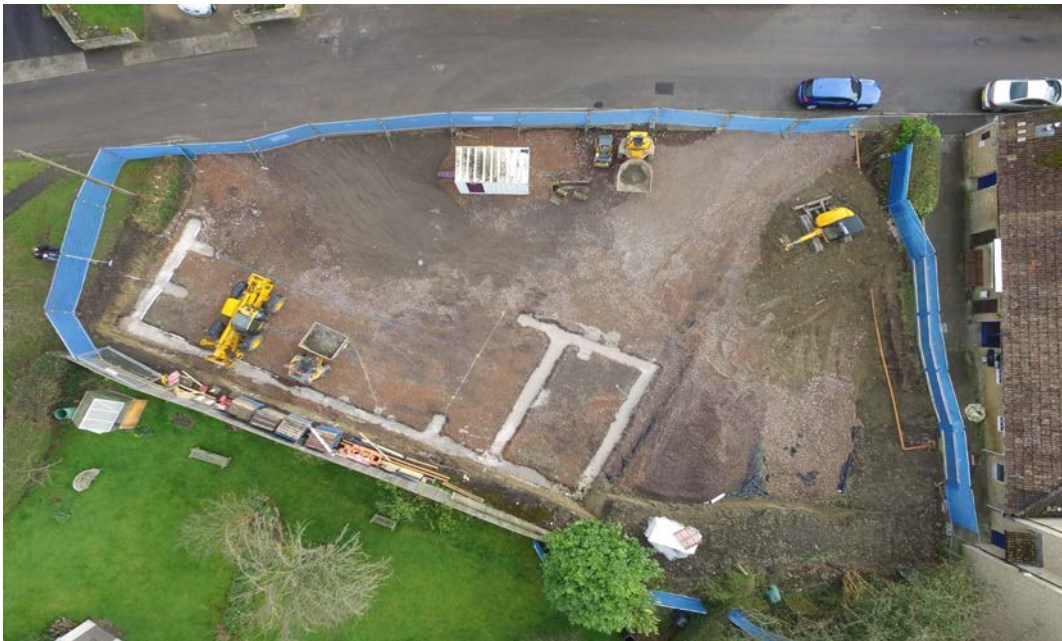
Photo. 3 Foundation Construction Underway
