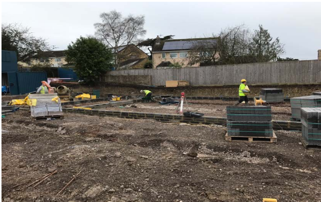
Photo 4 Masonry Construction underway
