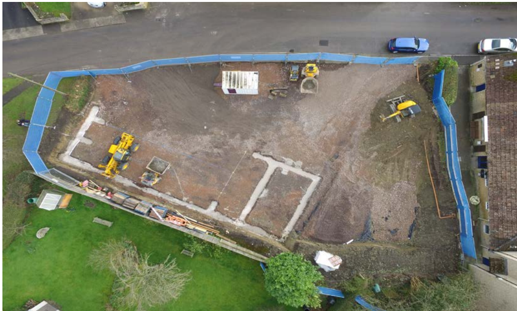
Photo. 3 Foundation Construction Underway
