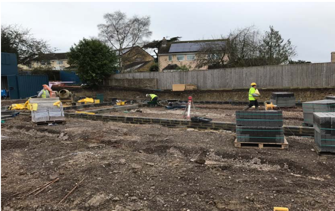
Photo 4 Masonry Construction underway
