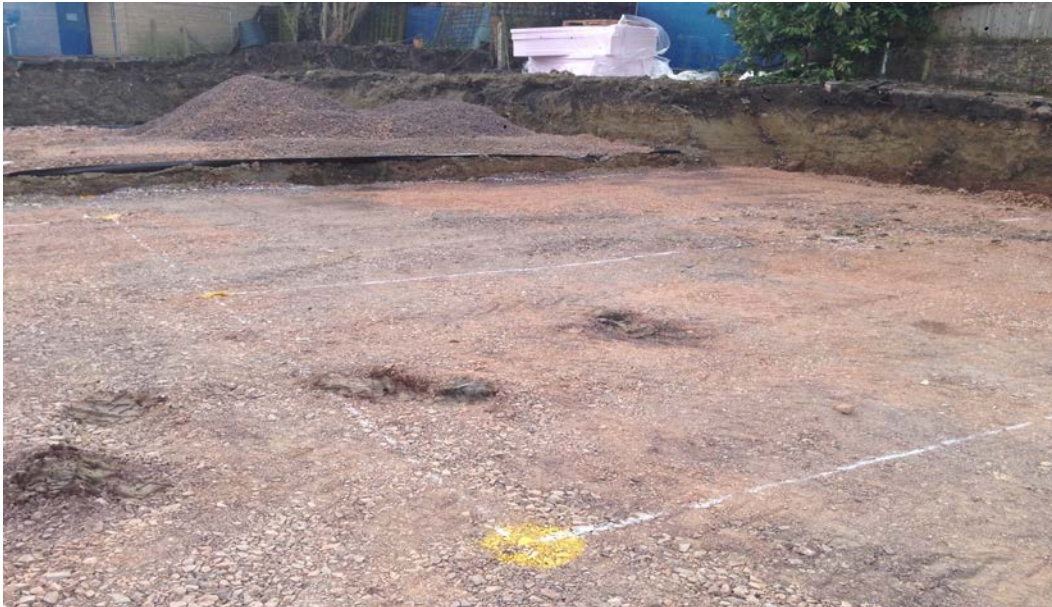
Photo 1. Foundation Setting out
