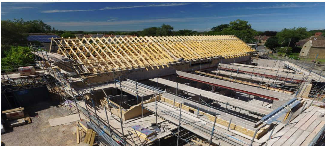
Photo 2. View across the building from over the site entrance
