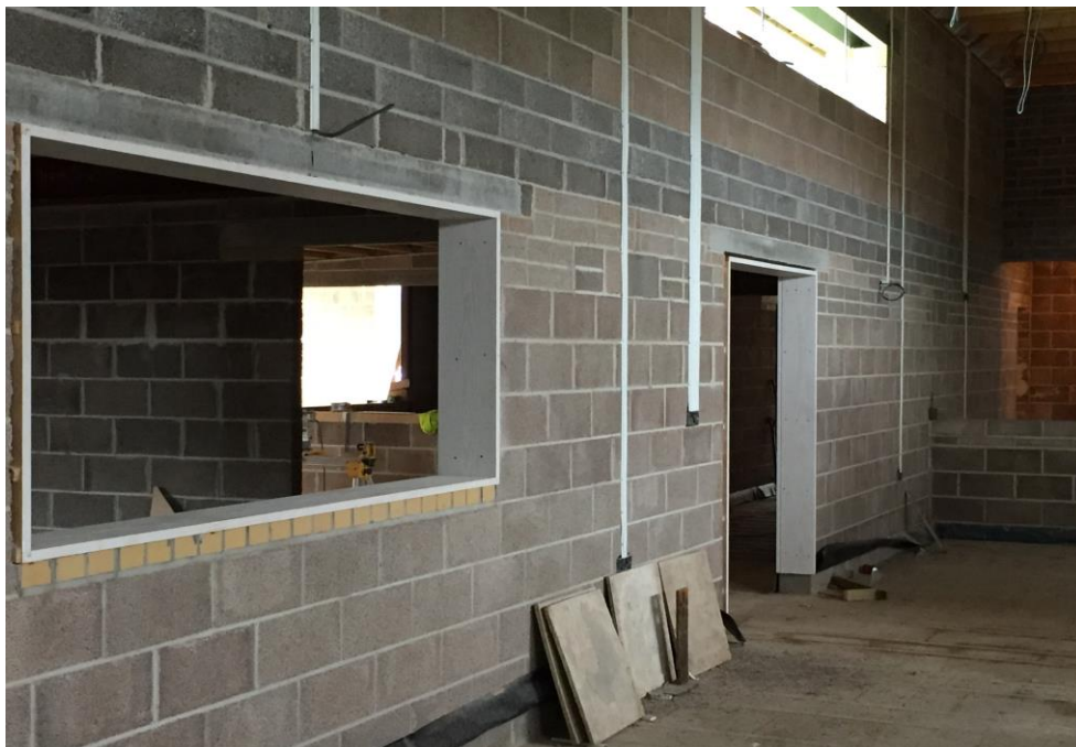
Picture 6. First fix electrical and door linings
