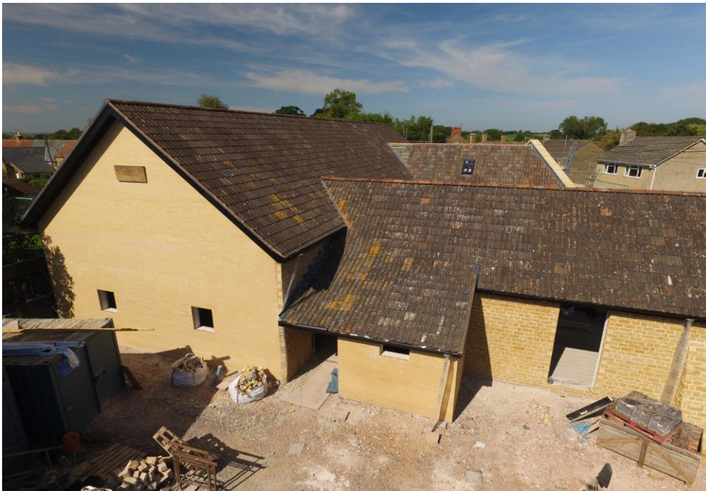
Picture 3. Carpark Elevation after scaffold removal
