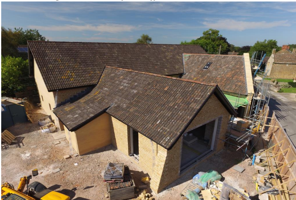
Picture 4. View from car park entrance after scaffold removal.
