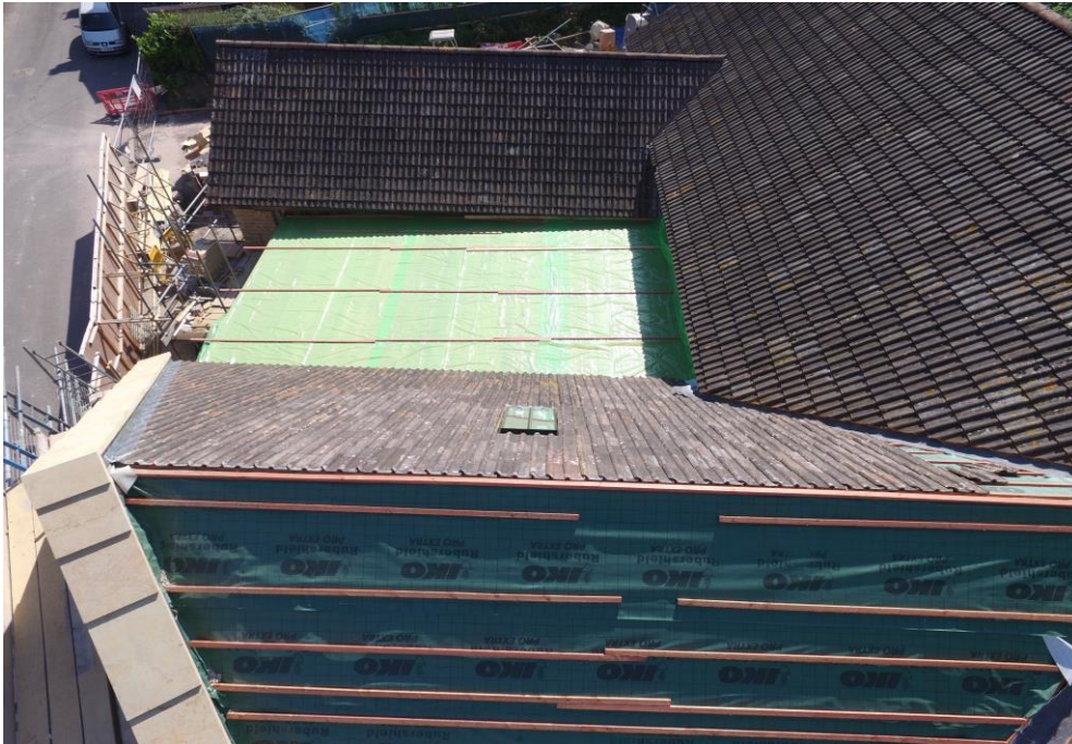
Picture 1 . Showing Roof Coverings
