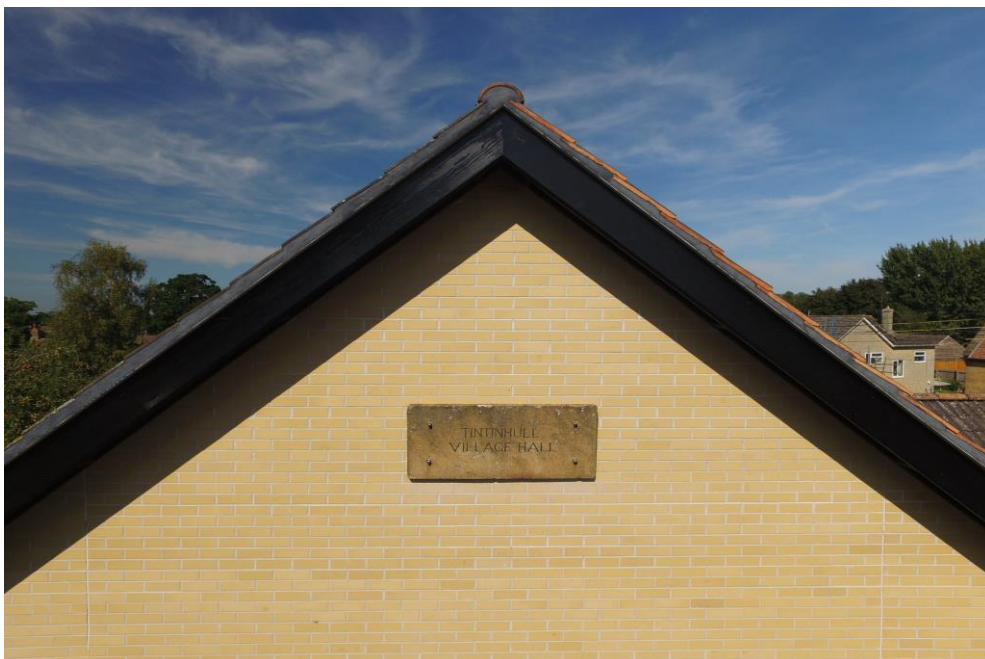
Picture 2. Reclaimed hall sign in position.
